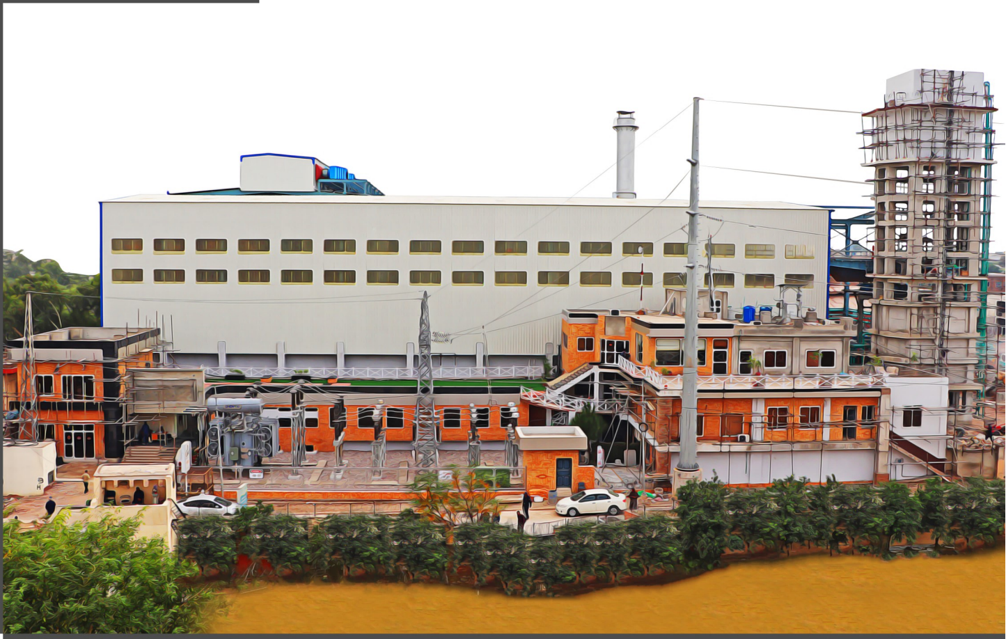
FF Unit-2 Peshawar after completion of 40 Mega Watt Grid, newly erected hanger for scrap, operational induction furnaces & CCM.
